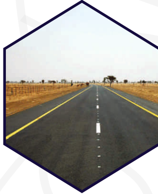
40' WIDE ENTRANCE ROAD
